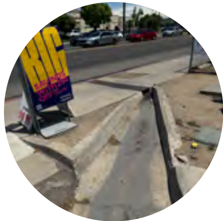
[Image above] Parking lot drainage at a local gas station which drains directly into local waterways
